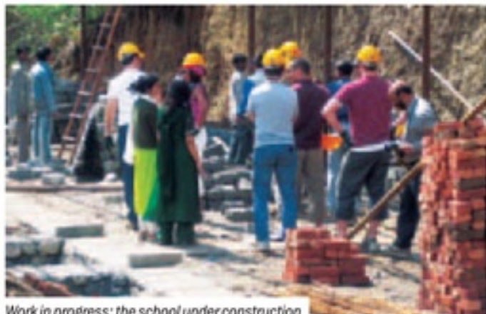
Work in progress: the school under construction
